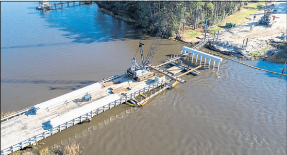
Steve Wingfield/Coastal Carolina Camera Club Replacement of the Calabash River bridge got underway earlier this year and work crews have now begun deconstructing the existing 48-year-old bridge. Shown are construction crews deconstructing the existing Calabash River bridge earlier this month. The contractor is taking the old bridge apart in pieces.
