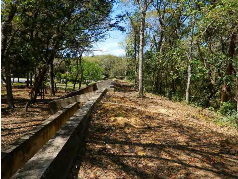
Photo A. Previously condition with removed vegetation.
