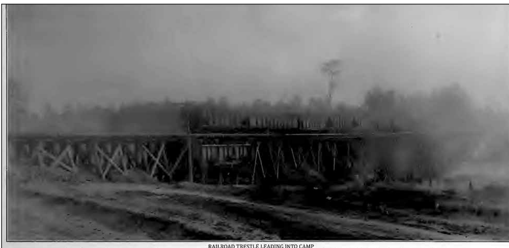
RAILROAD TRESTLE LEADING INTO CAMP
