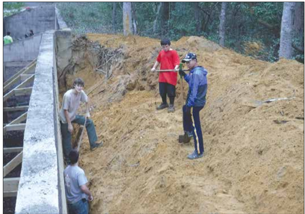
Terracing the back side of the fragile north wall
