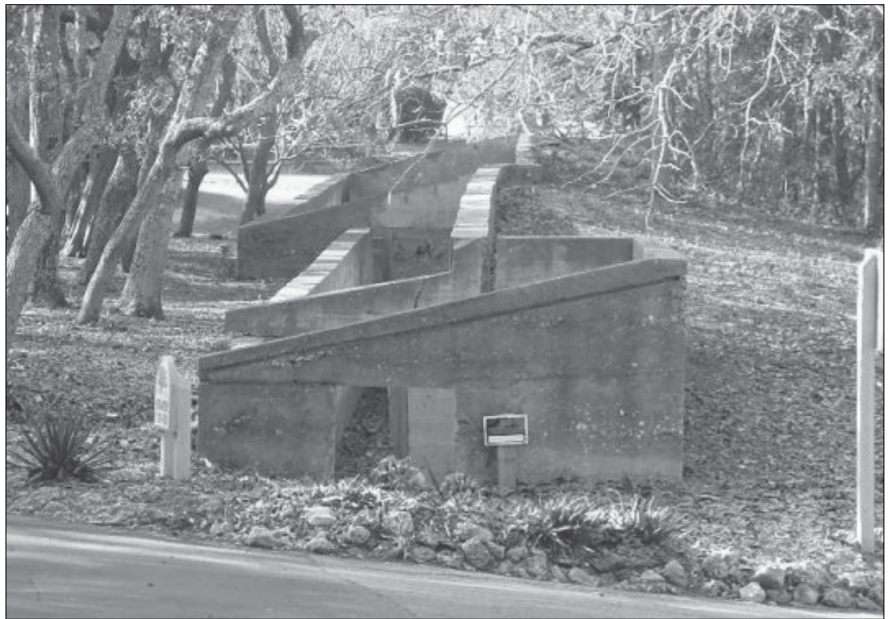
The 184-foot-long Fort Caswell Rifle Range wall is shown from the east side where the center wall is tilted inward displaying the need to stabilize it before it collapses.
