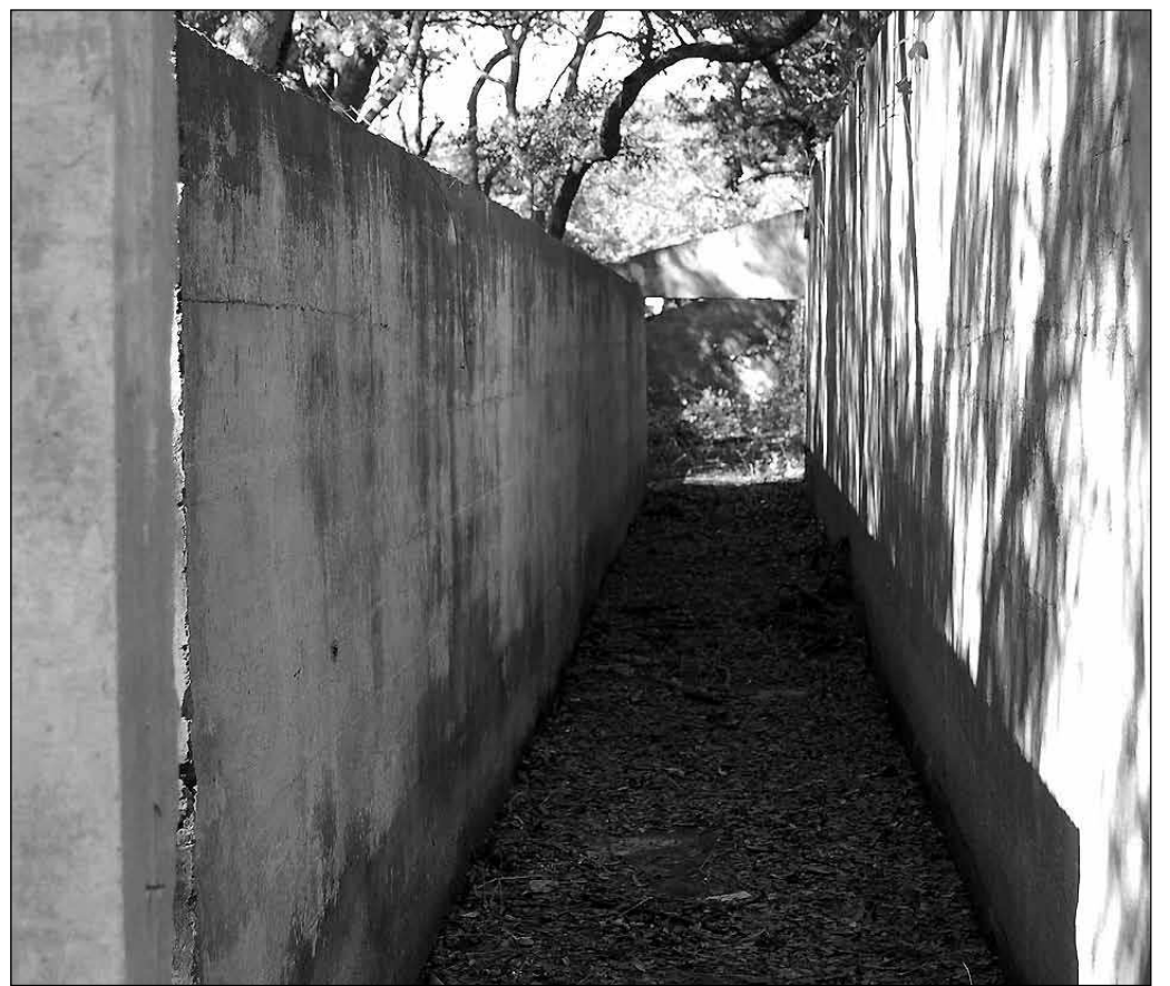
This view shows the long interior of the range, where targets were hoisted above the wall to the right.
